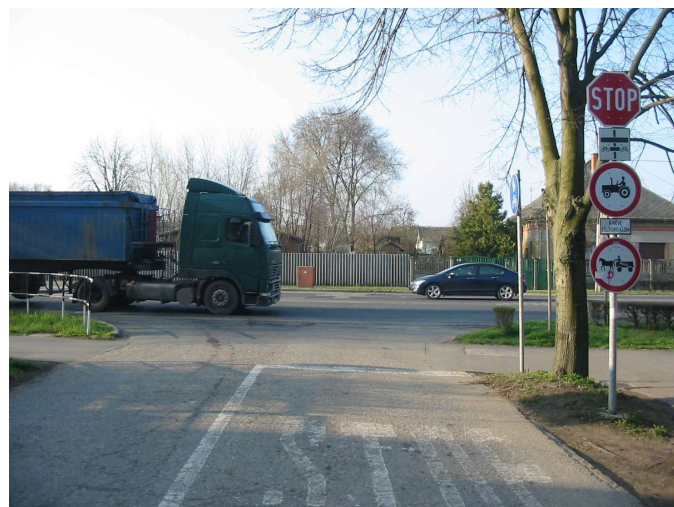
Fig. 3. Poor visibility of pavement markings at bicycle crossings [8]
